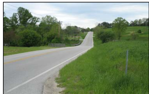
Typical lanes and shoulders along KY 715
