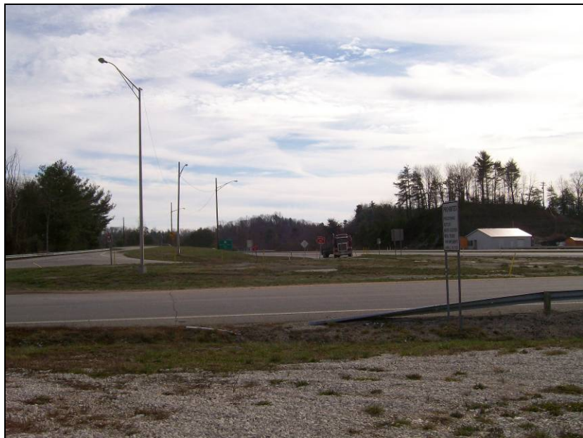
Mountain Parkway Exit 40 (eastbound ramps)
