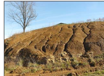
Residual Soil over Weathered Rock off Spencer Subdivision Road near Rogers
