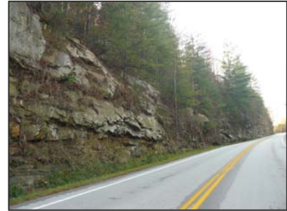
Rock Cut Slope along Southeastern Side of KY 11 near KY 715
