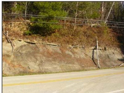
Cut Slope off KY 715 near Cliffview Resorts Road
