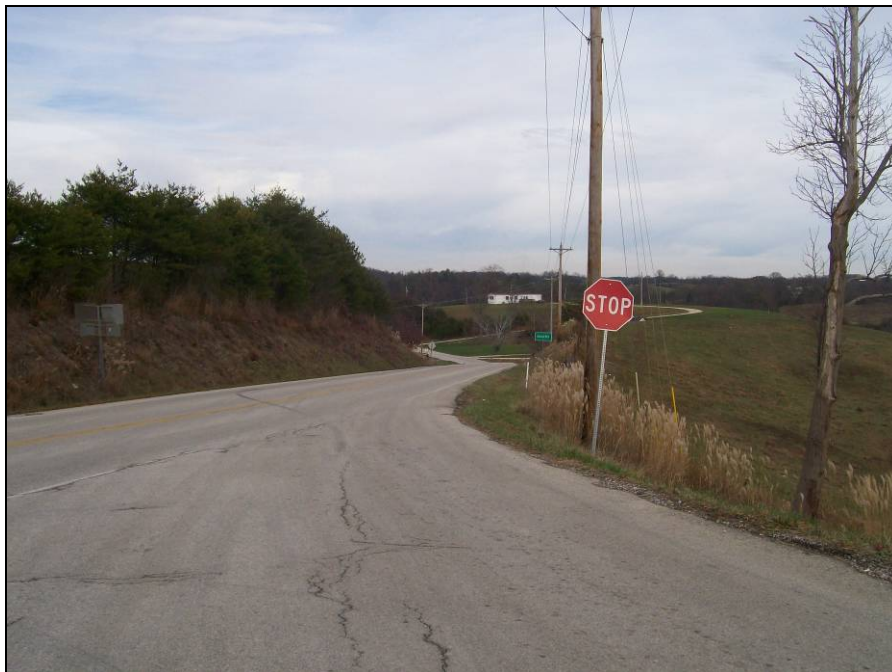
KY 2016 and KY 715 (northbound) Intersection
