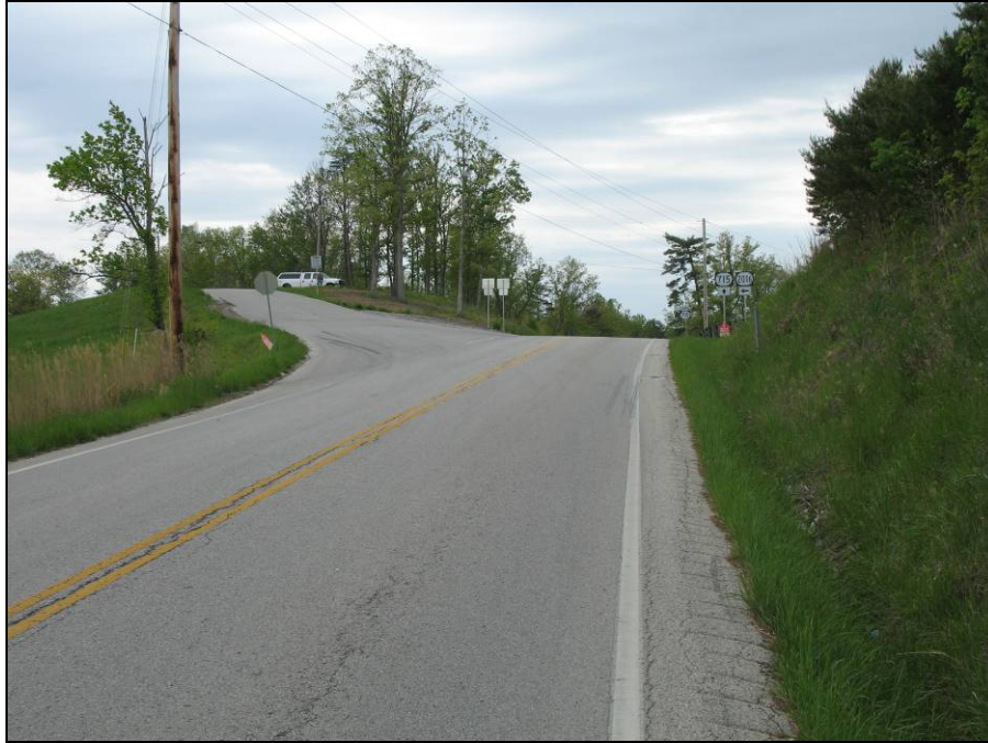
KY 715 (southbound) and KY 2016 Intersection
